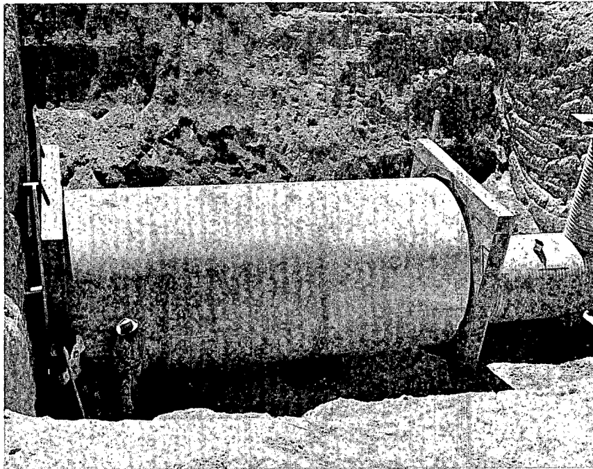
Figure 2.16 Exterior view of typical circular concrete conduit prior to backfilling.
